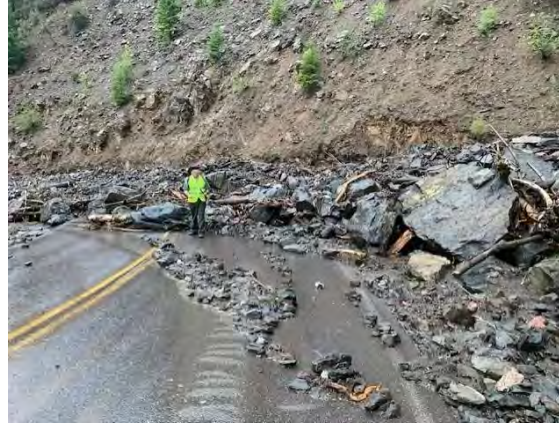
Debris flow at Curecanti National Recreation Area, July 16. From Black Canyon of the Gunnison National Park.
