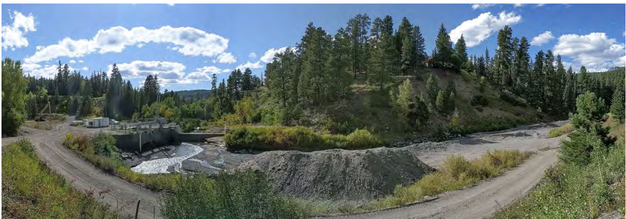
Figure 35. Evidence of sediment removal activities (image-center) on the upstream side of the Blanco Diversion Dam on the Rio Blanco.
